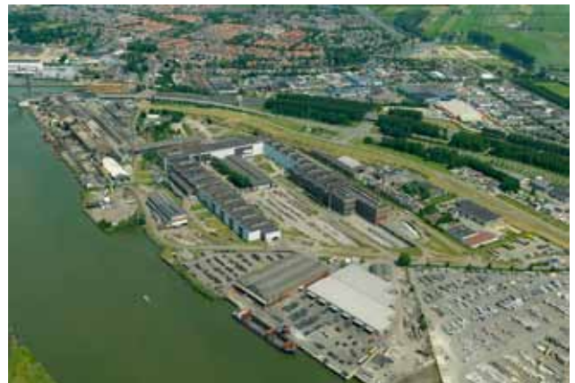
棒材厂和线材加工中心，阿尔布拉瑟丹，荷兰 Rod Mill and Wire Processing Centre, Alblasserdam, The Netherlands
