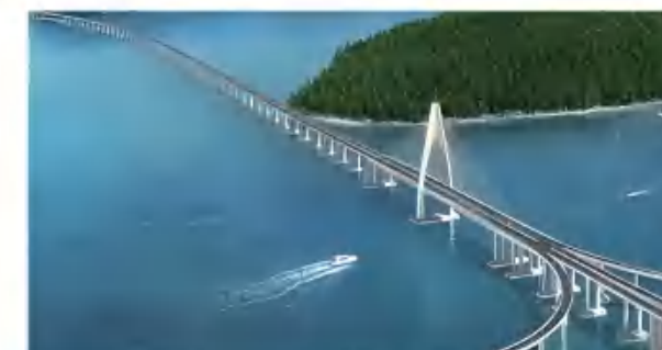
文莱跨海大桥 Brunei Sea-crossing Bridge
