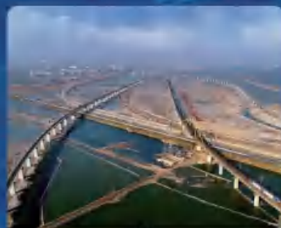
迁曹铁路 Qian'an-Caofeldian Railway
