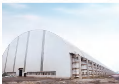
全封闭料场 Fully-Enclosed Stockyard
